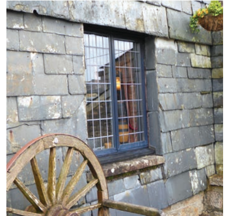
The slate-hung walls of Jamaica Inn, which, at the time that John Broad built his new house, was a distinctively Cornish style of building.
